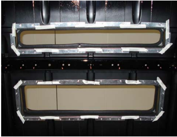
Figure 2-18 Preparation of Sikaflex application
