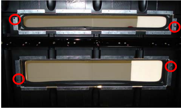
Figure 2-13 Transition Ducts (Interior)
