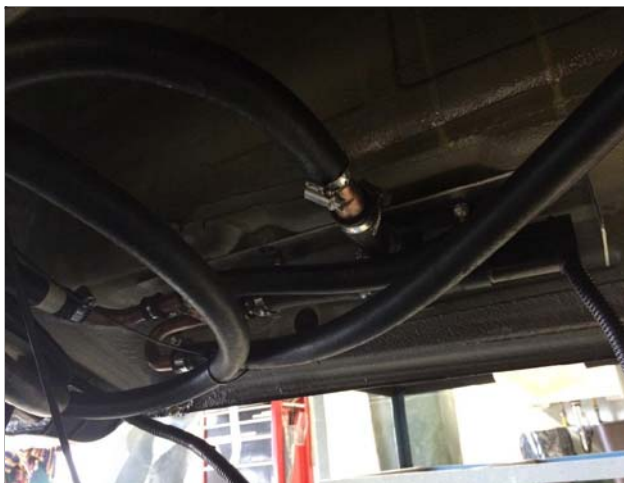
Figure 2-79 Heater Hoses Installed at Boost Pump
