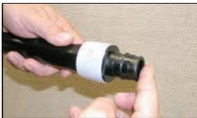
3. Insert coupling. The PEX pipe will contract and create a tight connection. (Allow one hour for PEX pipe to set before pressure testing.)
