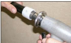
2. Expand the PEX pipe with the hydraulic expanding tool
